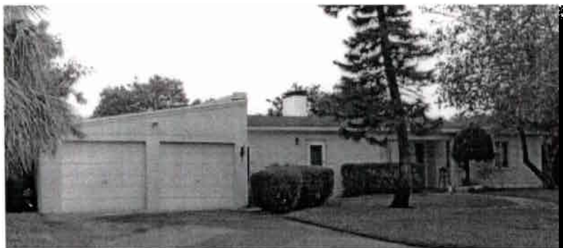
Inappropriate: Garage roof is not the same shape as the house
