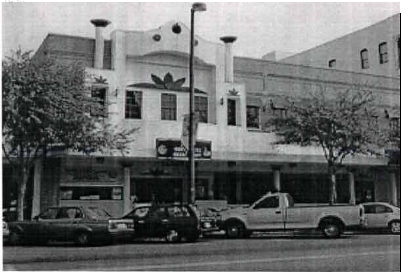
Inappropriate: False façade is added that is not in keeping with the architecture of the structure. Street level appearance is partially in keeping with the storefront/window display character.
