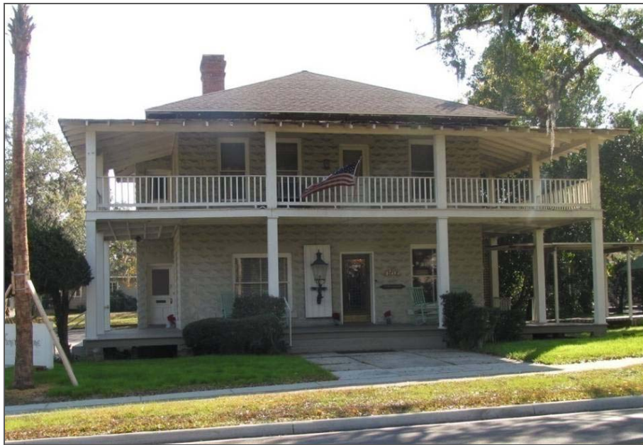
Figure 46: Early example of a Masonry Vernacular building constructed as a residence out of rusticated concrete block, now converted to commercial use at 456 E. Tarpon Avenue (8P11672)
