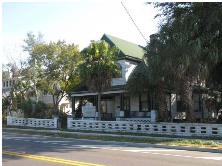
Figure 84: Rusticated block site wall along Tarpon Avenue (porch piers and foundations walls of the house behind are also constructed of rusticated block)
