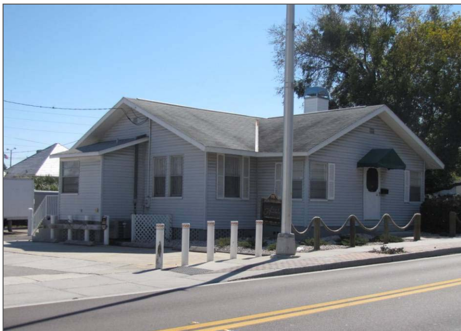
Figure 86: Historic home with porch enclosed, windows replaced and replacement siding
