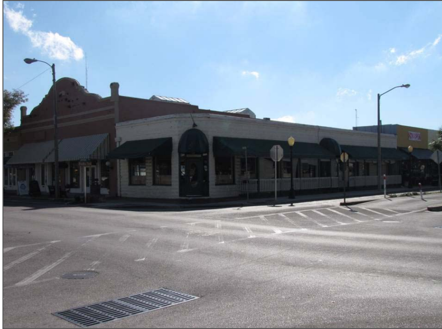
Figure 47: One-story Masonry Vernacular commercial building constructed of rusticated concrete block at 200 E. Tarpon Avenue (8PI1653)
