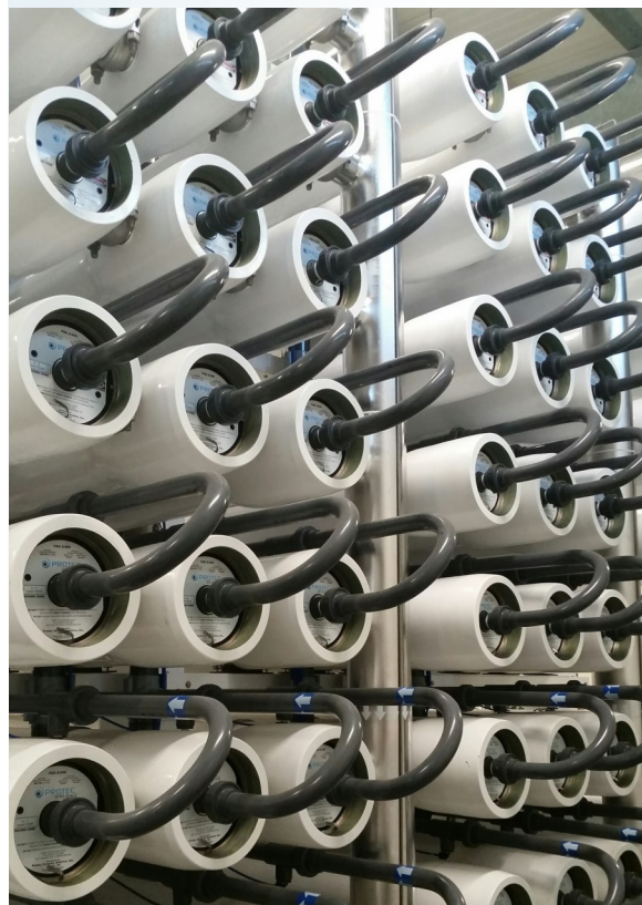
Reverse Osmosis Membrane Vessels at the City of Tarpon Springs Reverse Osmosis Water Facility
