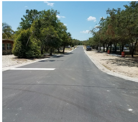
Final Paving from Lake Tarpon Sewer Project
