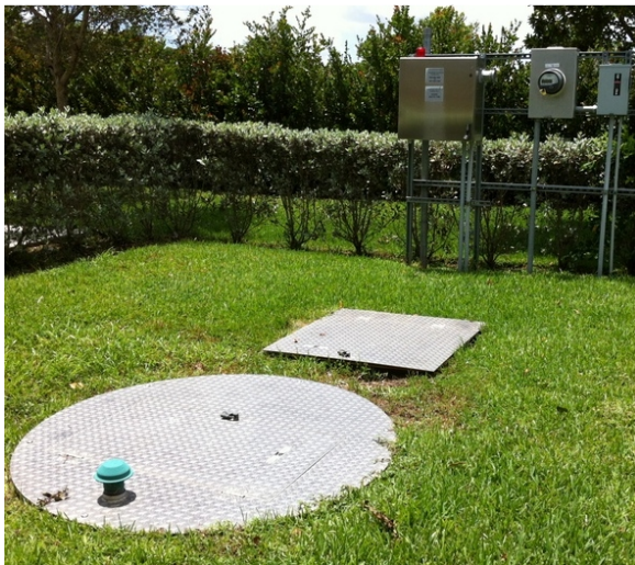
Lift Station Example
