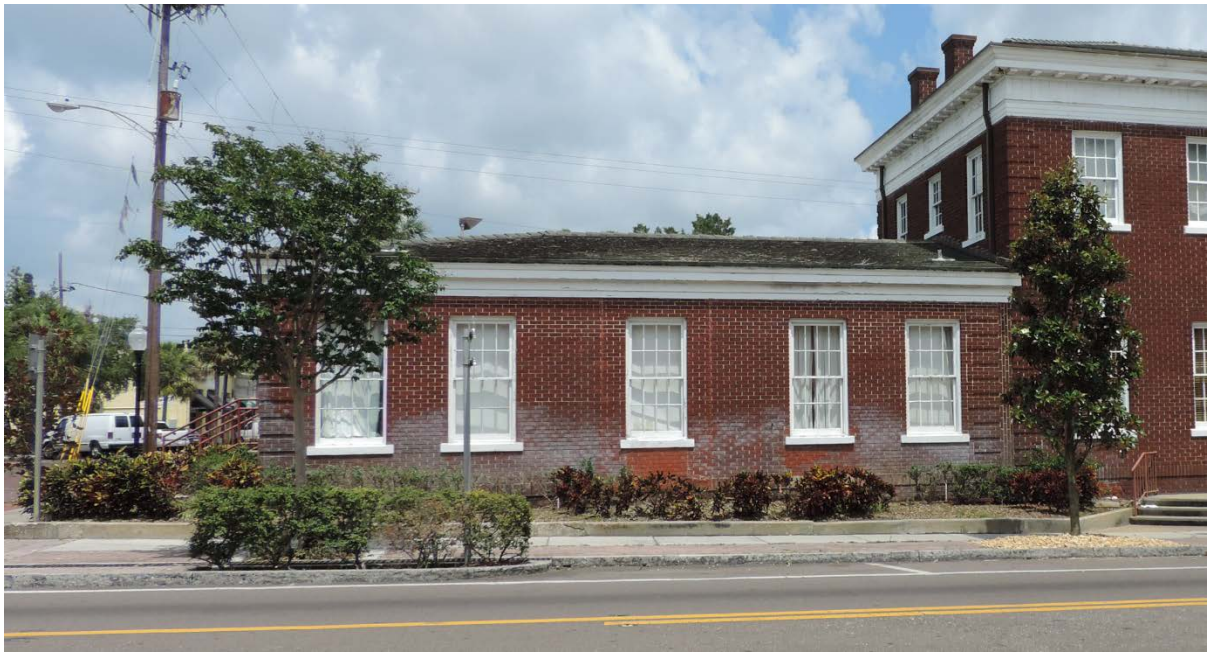
Photo 6: West Elevation – one story addition
