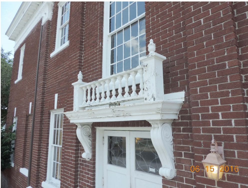
Photo 10: East entrance door hood with balustrade above
