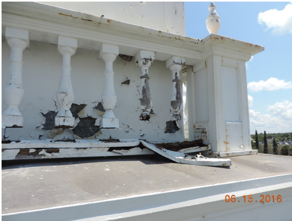
Photo 14: Clock tower balustrade
