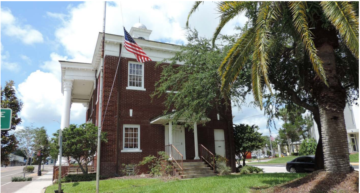
Photo 2: South Elevation – Looking northeast
