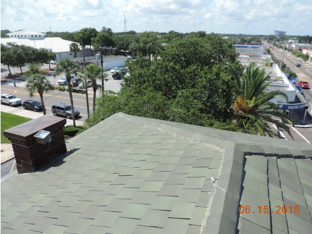
Photo 17: Hip and ridge tiles at roof, looking southeast
