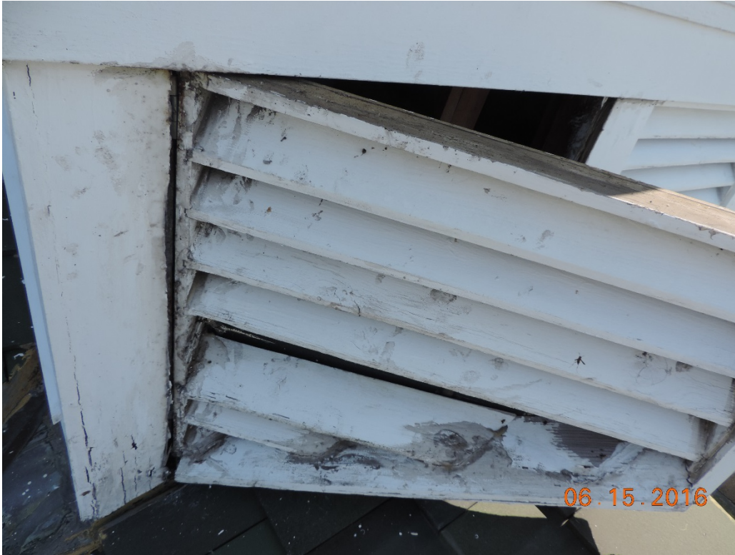
Photo 15: Clock tower hinged louver access door
