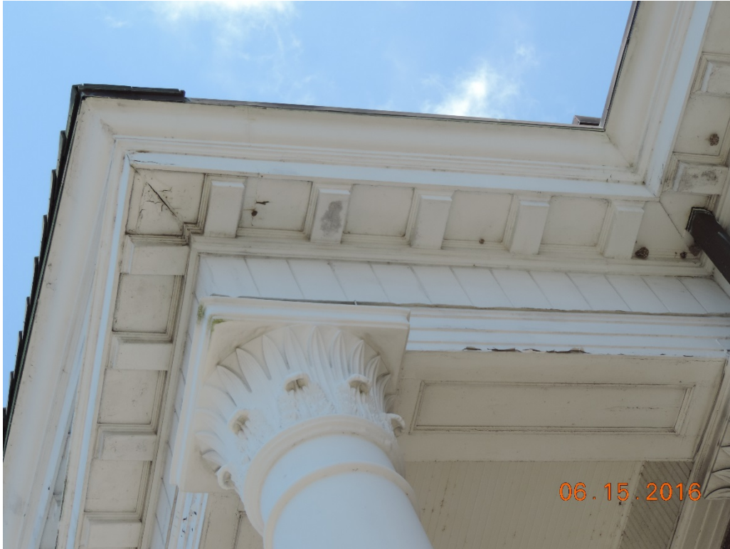
Photo 7: Cornice at front two-story portico – column capital, wood ceiling and trim
