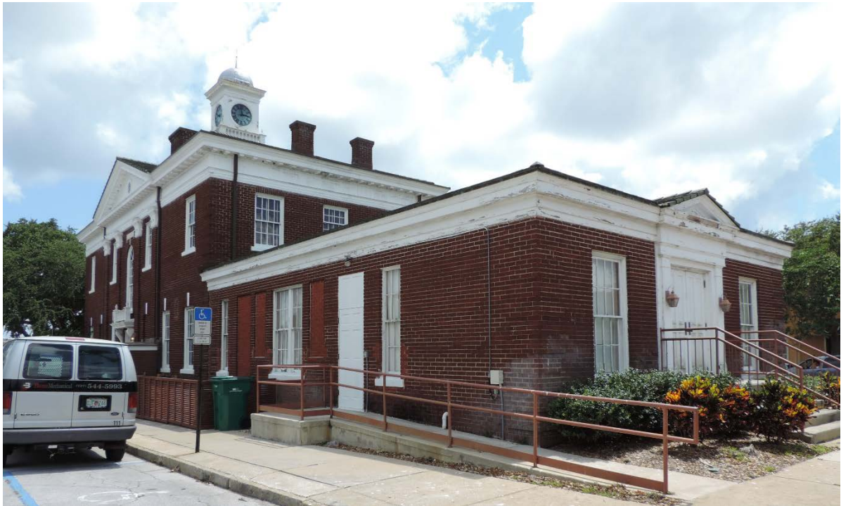
Photo 5: North and East Elevations – one story addition
