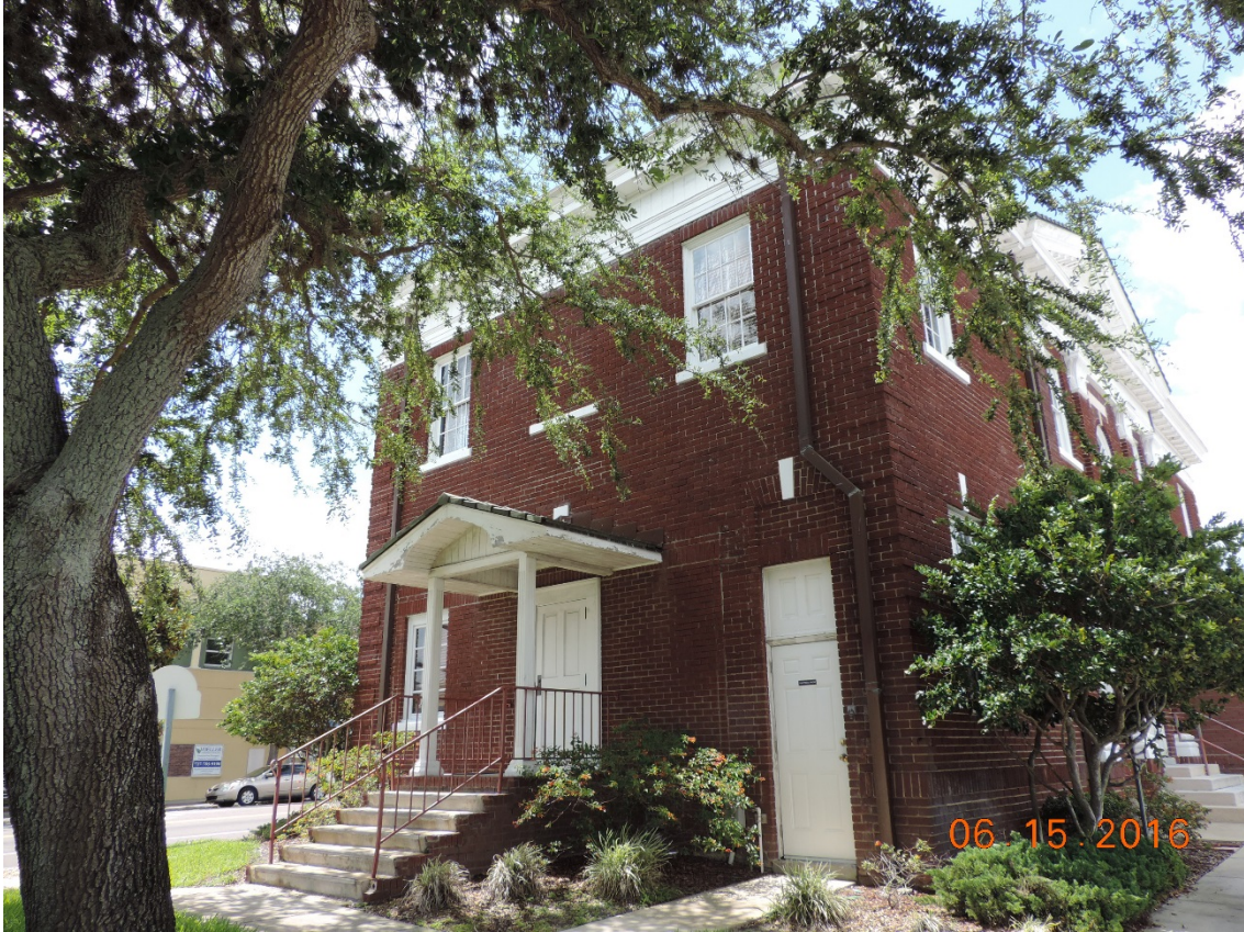
Photo 3: South Elevation – Looking northwest
