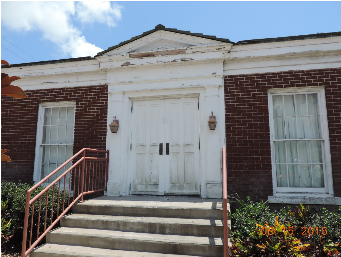
Photo 12: North entrance at one story addition, rotted woodwork to be replaced to match existing.
