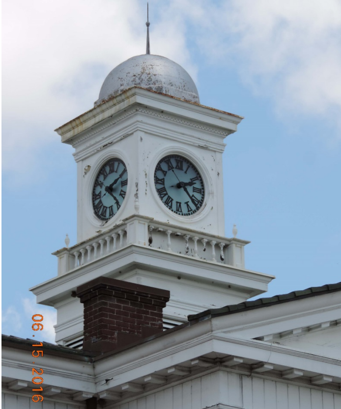
Photo 13: Clock tower with balustrade, capped chimney, main building cornice, looking southeast
