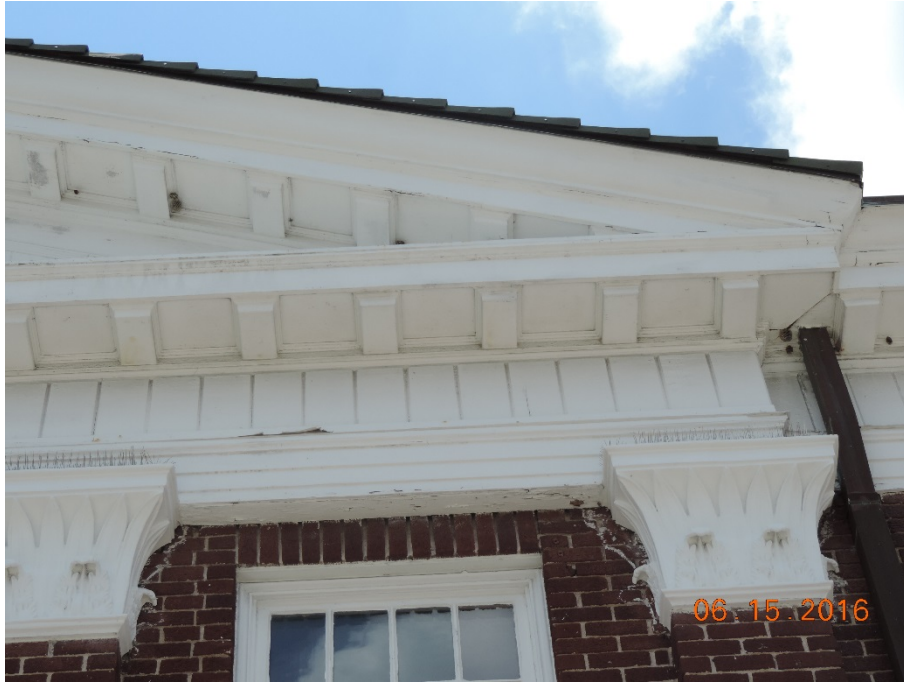
Photo 11: Cornice, pilasters capitals, and pediment at east elevation
