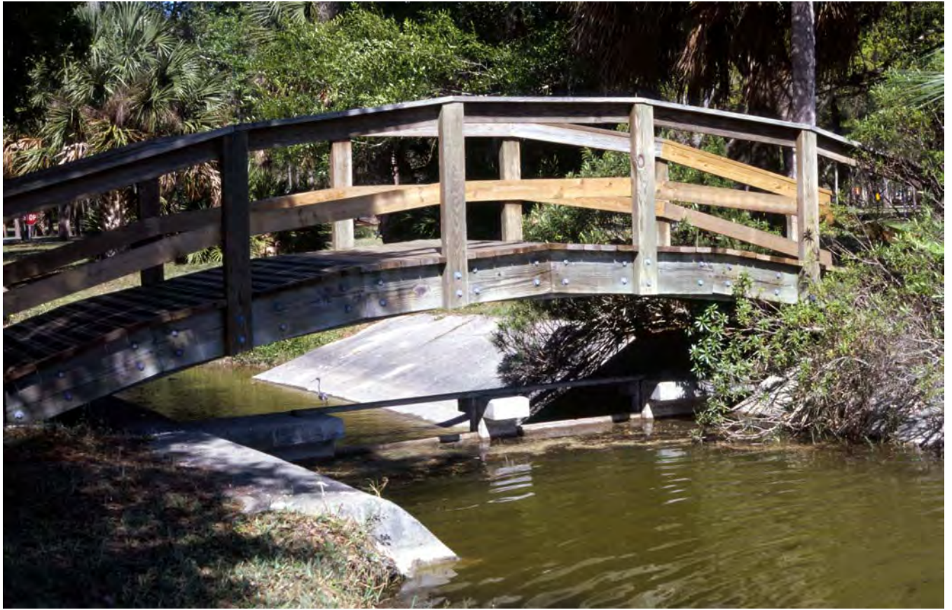
Figure 14.—A concrete water-control structure that minimizes erosion and controls the water level in a small lake.
