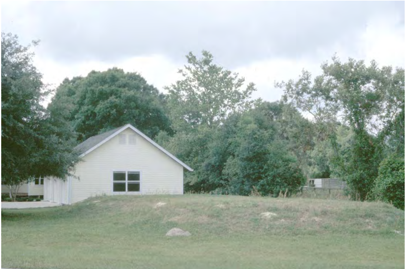
Figure 15.—An area of Felda fine sand in which a septic system has been placed in a raised bed due to a seasonal high water table.
