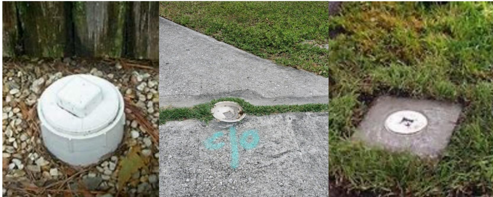
These are sewer clean out pipes. They provide access to the lateral line that connects your home to the public sewer line. Clean outs allow clearance of your line and reduce the need to call a plumber or further damage from a sewer backup. It is important to keep these clean outs clear and unobstructed to allow for quick access to clear clogs.
