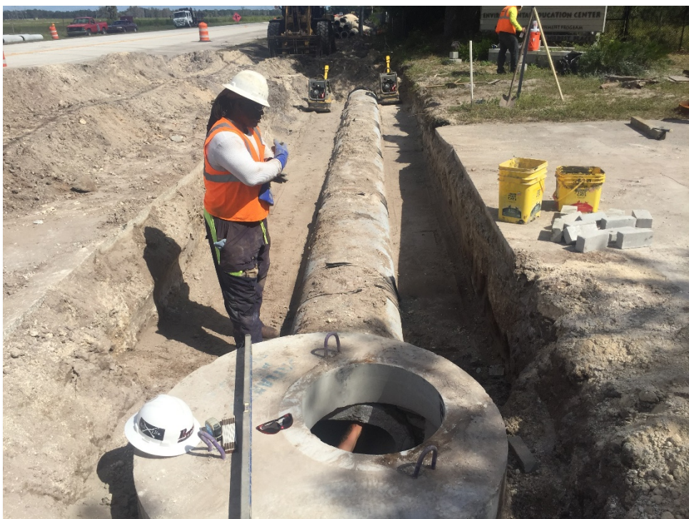
Stormwater manhole and pipe
