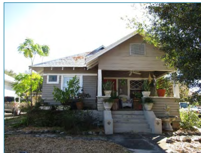
Figure 117: Exposed rafter tails on 31 Read Street should be maintained and not removed or enclosed.
