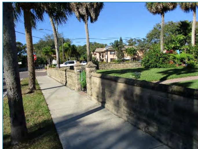
Figure 88: A natural reticulated block wall at 36 North Spring Boulevard.
