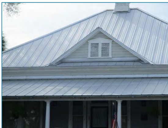
Figure 113: A replacement standing seam metal roof on 412 East Tarpon Avenue.
