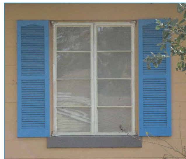
Figure 107: Two examples of shutters that are decorative but not functional. They are not large enough to cover the entire window when closed and are therefore do not follow the guidelines.
