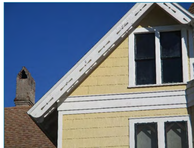
Figure 77: The dwelling at 22 North Spring Blvd is clad in 20th-century asbestos shingles.
