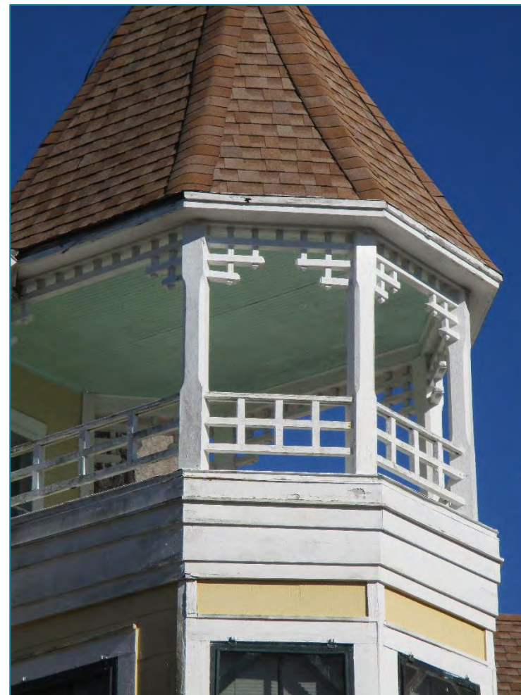
Figure 73: The wood trim on this balcony displays peeling paint and some damaged wood. Architectural features should be preserved rather than replaced.
