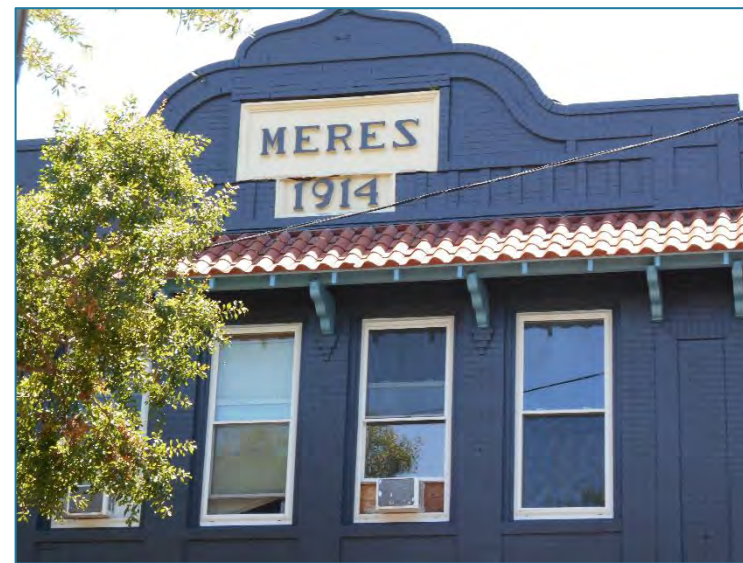
Figure 125: Replacement windows on the second floor of the Meres Building match the historic window openings and type but not material.
