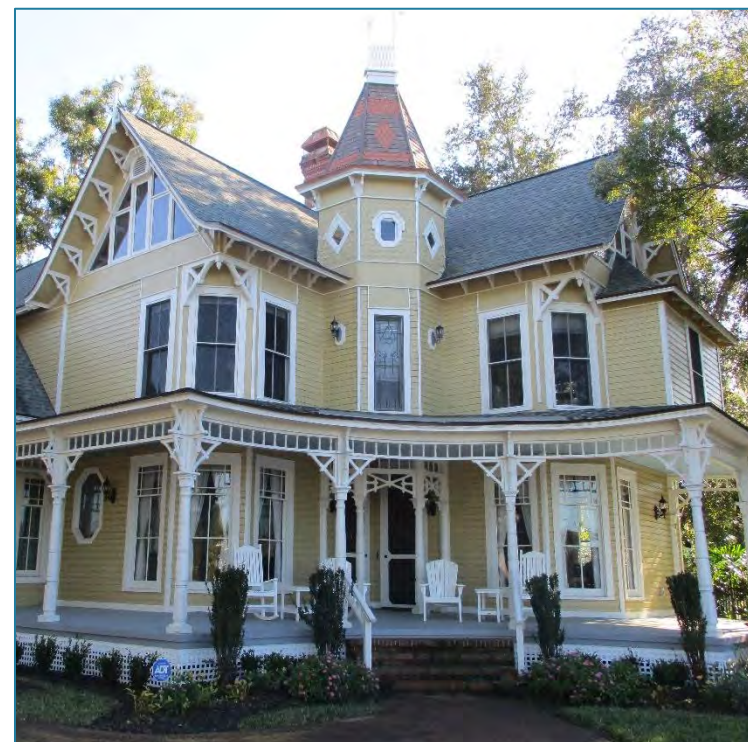
Figure 74: This well-preserved dwelling at 115 S Spring Boulevard retains significant historic features such as original windows, masonry chimney, and carved wood bracketry and porch details that should be restored rather than replaced.
