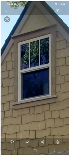
Proposed window; PGT Impact vinyl frame white with vertical muttons. The mutton count will vary depending on window width but will match existing very closely. Window trim will not change style. It may be repaired or replaced with the same material and profile if decayed or damaged when window is replaced.
