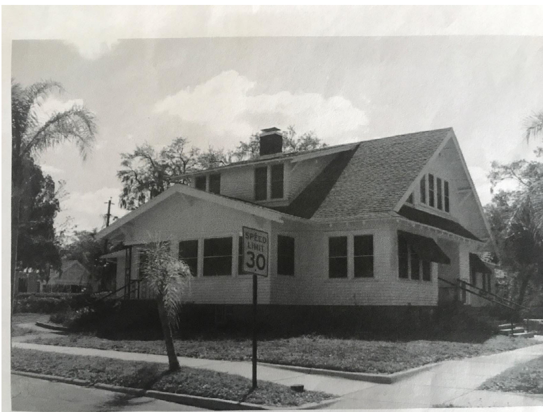
1980's photo. notice windows, roof change, stair change.
