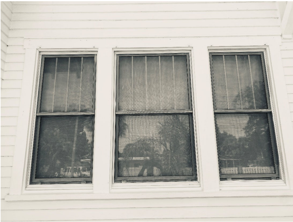
2020 photo of original windows from the 1960's.
