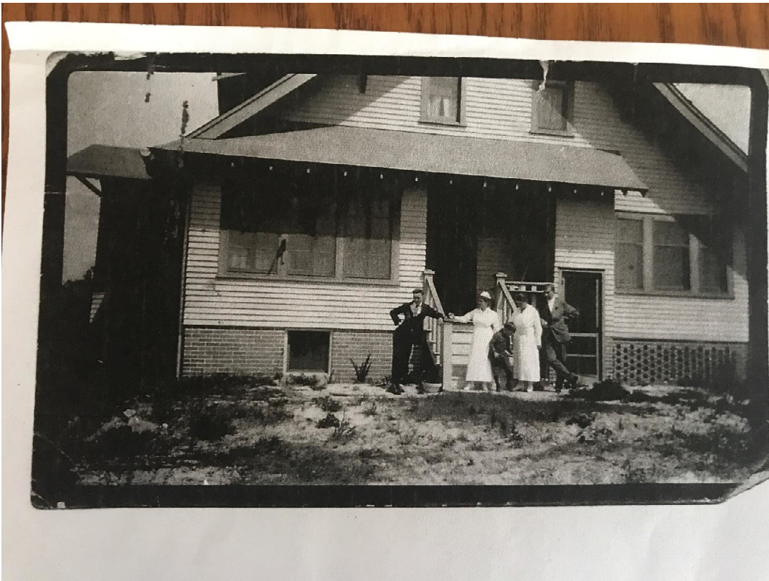
Photo from 1915. Notice the metal roof, stair & banister rail, exposed rafter tails.
