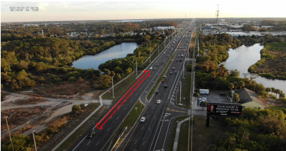
Figure 5: Example of 5 Second Gap (Looking Southbound)
