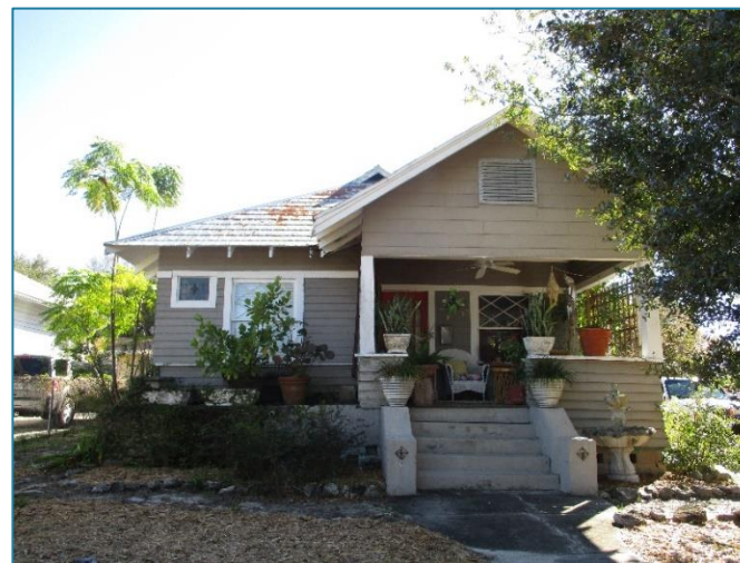
Figure 118: Exposed rafter tails on 31 Read Street should be maintained and not removed or enclosed.
