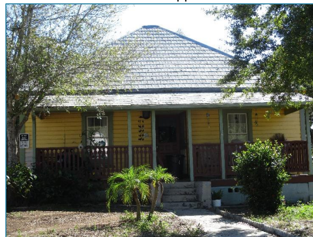
Figure 27: Example of a one-story Frame Vernacular residence with a rectangular plan, hipped roof and shed roof porch at 73 Park Street.
