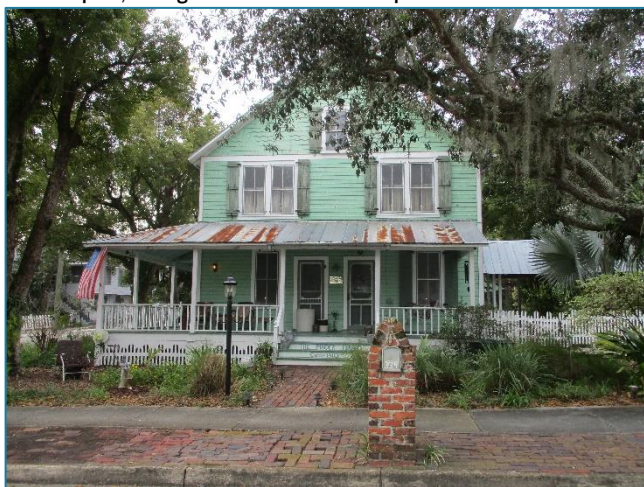
Figure 26: Example of a two-story Frame Vernacular residence with a rectangular plan, front gable roof and porch that wraps three sides at 344 E Orange Street.
