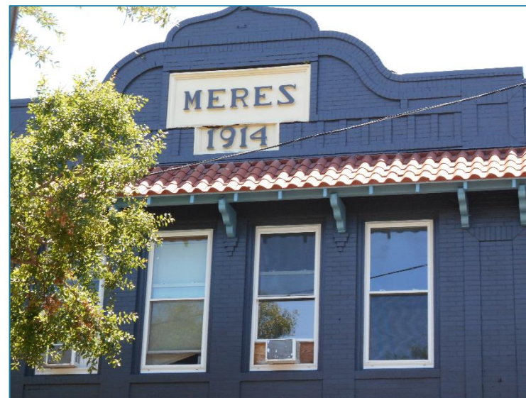
Figure 126: Replacement windows on the second floor of the Meres Building match the historic window openings and type but not material.
