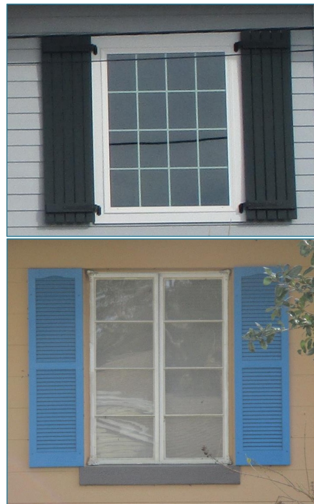
Figure 108: Two examples of shutters that are decorative but not functional. They are not large enough to cover the entire window when closed and therefore do not follow the guidelines.
