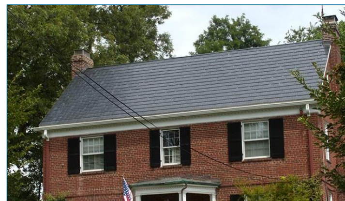
Figure 102: Historic home with solar shingles. Photo source: https://www.nps.gov/tps/standards/rehabilitation/guidelines/roofs.htm
