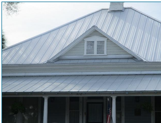
Figure 114: A replacement standing seam metal roof on 412 East Tarpon Avenue.
