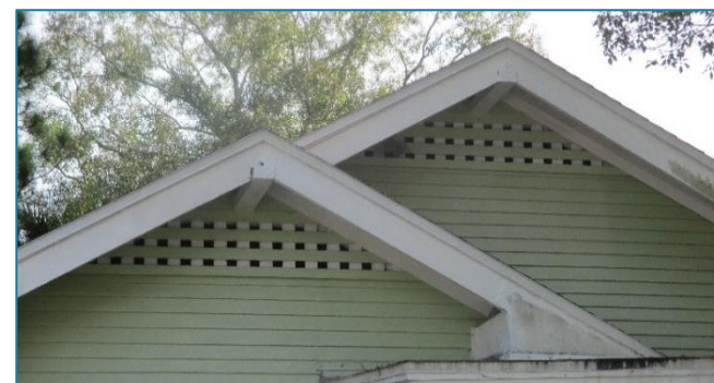
Figure 104: Architectural details are used to create gable vents on 225 Pineapple Street.
