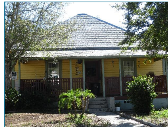
Figure 115: A metal shingle roof on 73 Park Street.
