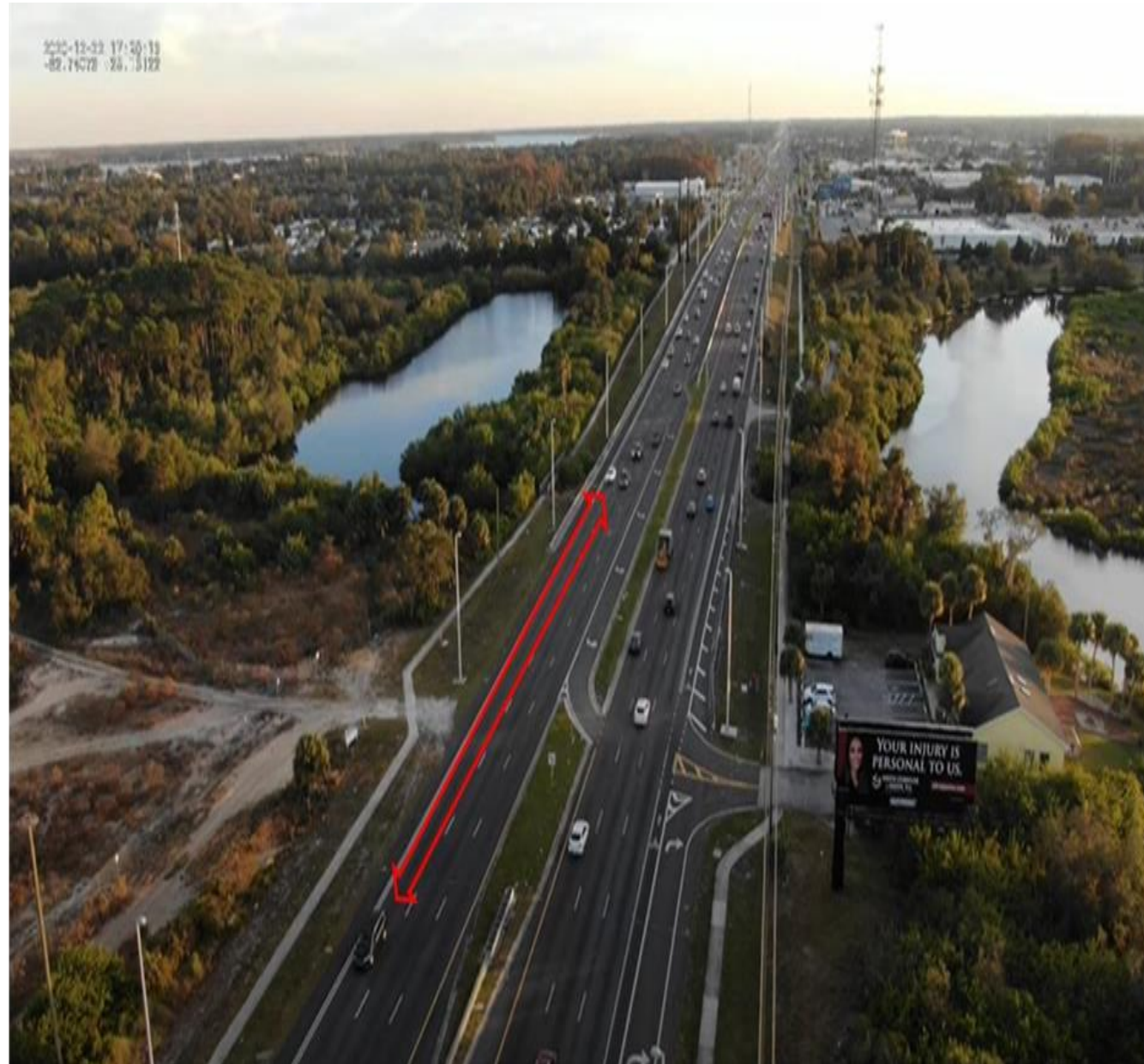
Example of 5 Second Gap (Looking Southbound on US 19)
