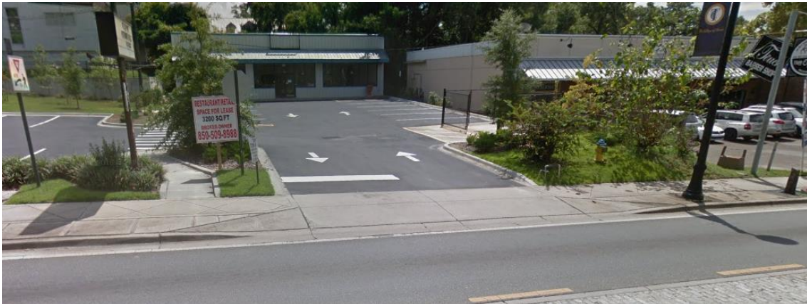
Figure 38 – Flared Driveway Example
