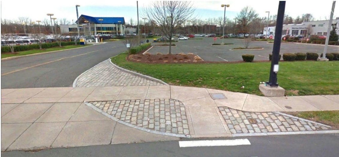
Figure 87 – Truck Apron and Driveways
