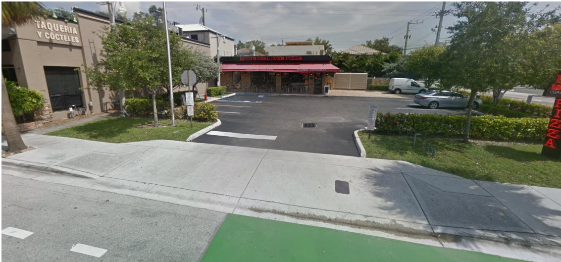
Figure 7 – Curbed Roadway (Flared Return)
