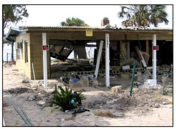
Figure 2. Masonry walls destroyed by 3 feet of stillwater flooding and small waves (Hurricane Dennis).
