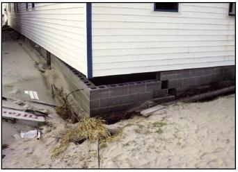
Figure 4. Failure of A Zone type foundation in coastal area, not subject to V Zone conditions (Hurricane Fran).
