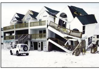
Figure 1. Failure of wood-frame walls used to support a coastal building, which was subjected to shallow flooding, small waves, and floating debris (Hurricane Opal).
