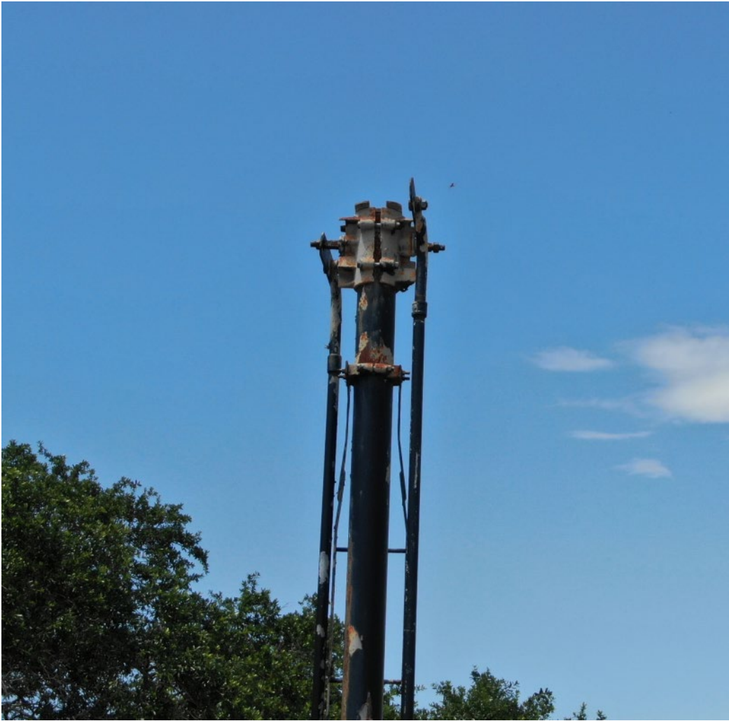
City's Existing Signal Mast, view from the ground
