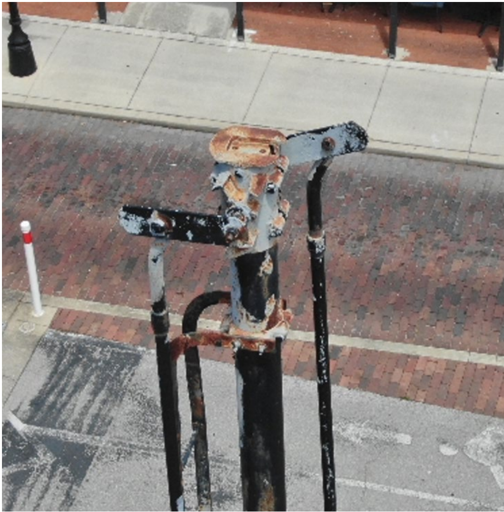
City's Existing Signal Mast, view from the top
