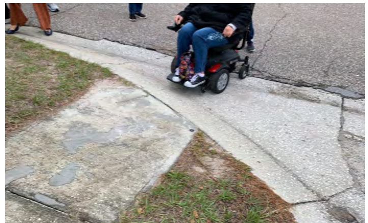
Non-ADA compliant curb ramps along Disston Avenue.
