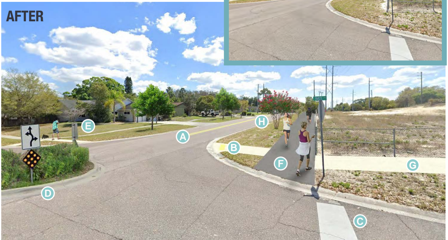
Location: Disston Avenue and Ivey Lane looking south.
