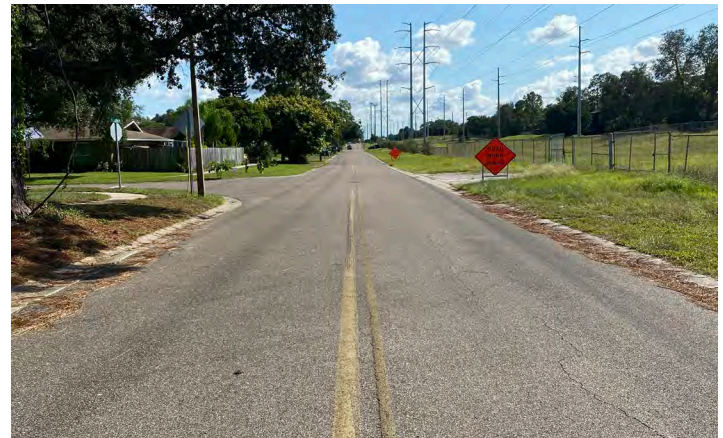
Disston Avenue facing south near Sugar Mill Road.
