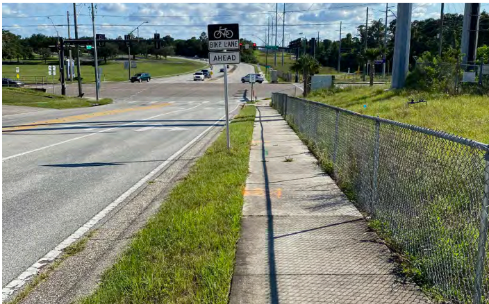
Sidewalk on west side of Disston Avenue near Klosterman Road.
