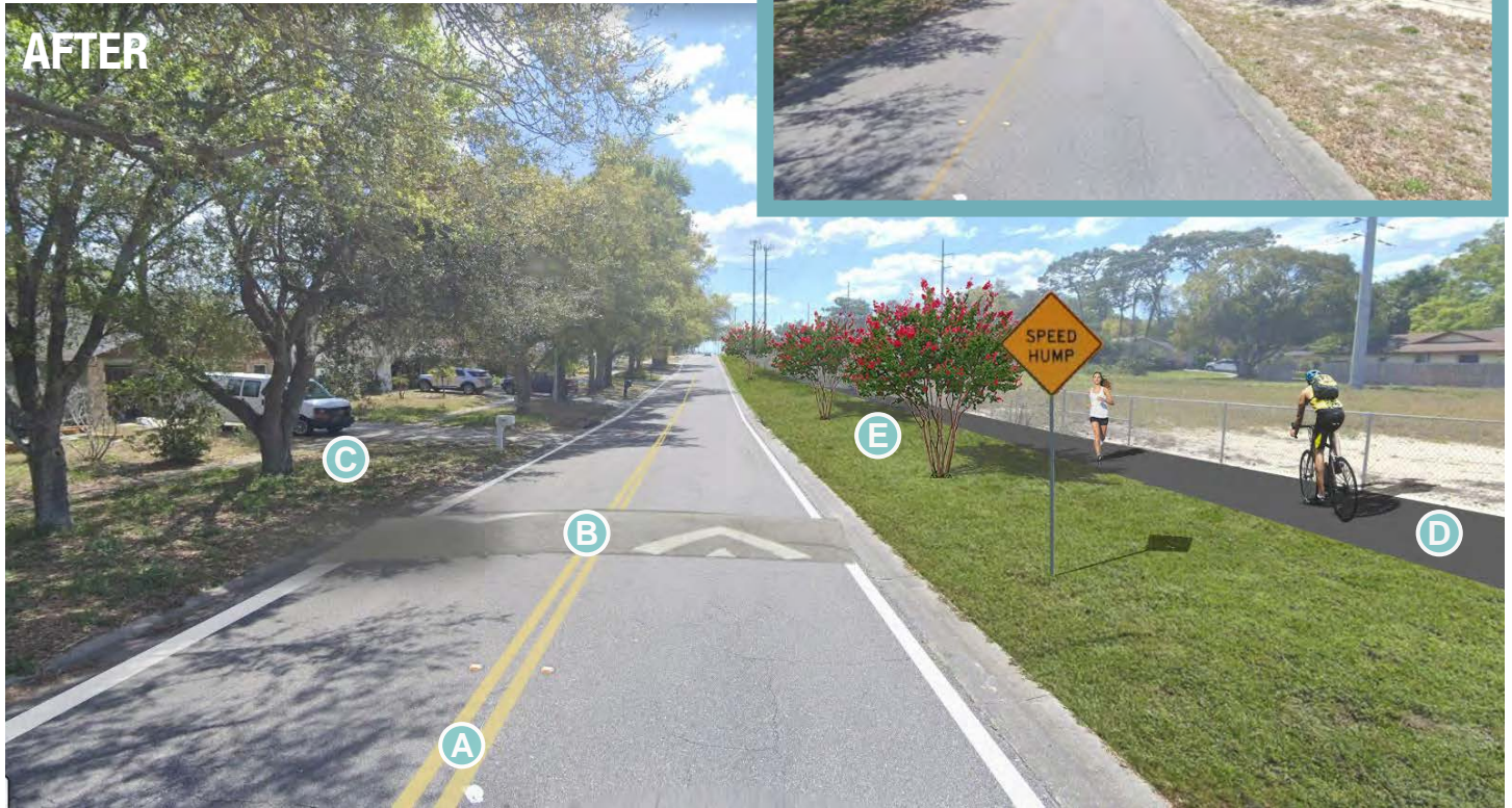
Location: Disston Avenue between Ivey Lane and Sandy Hollow Road looking south.
