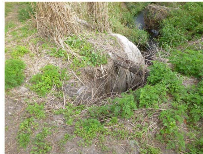
Figure 1 Outfall facing southeast.
