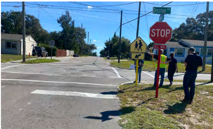
Non-standard signage at Disston Avenue and Pent Street intersection.
