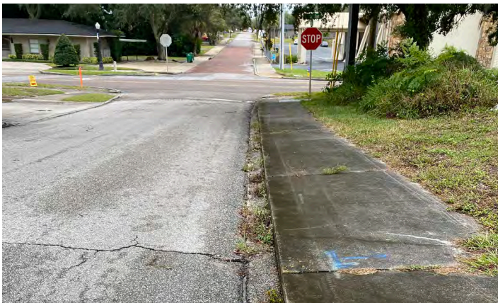
Sidewalk on west side of Disston Avenue near Tarpon Avenue.
