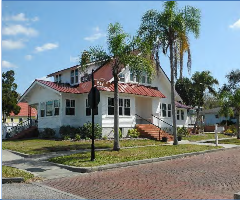
Figure 43. The home at 201 Bay Street is elevated on a continuous brick foundation wall and includes a basement. The elevation well above grade is emphasized by the long staircases leading into the front and sides of the structure.
