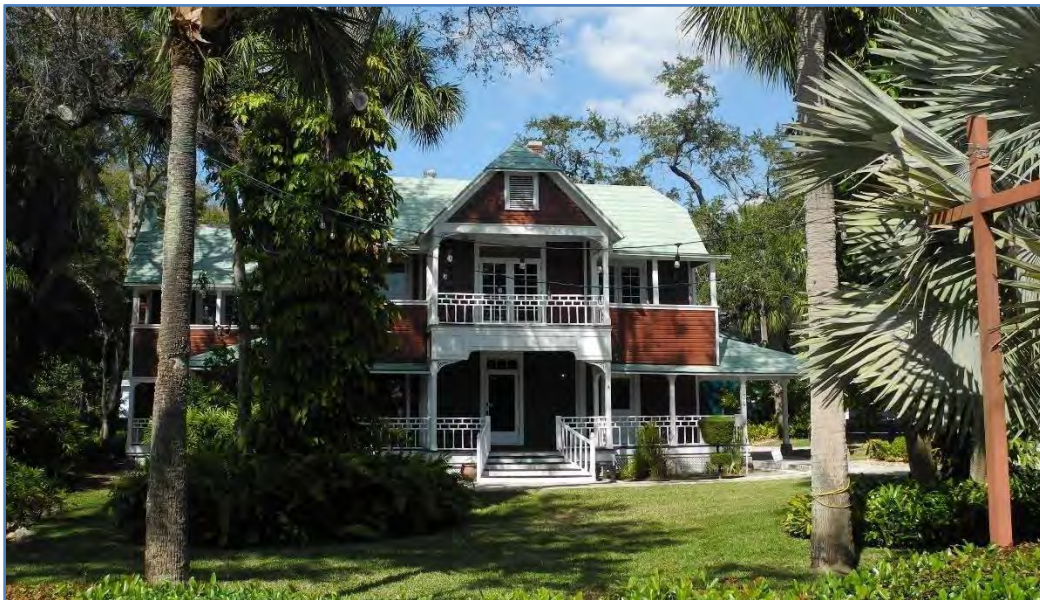
Figure 15. Frame Vernacular style house on crawl space with lattice infill, 2022 photo.
