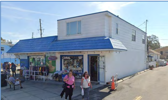
Figure 48. The structure at 805 Dodecanese Boulevard is a mixed use building designed to place living area on the second floor above the expected flood elevation. This approach can include permanent floodproofing measures or temporary protective floodgates and flood-wrapping, as illustrated.
